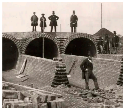
Bazalgette inspecting work on new sewage tunnels.
