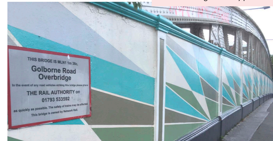
Below: The RBK&C Goldborne Road Overbridge is freshly painted.
