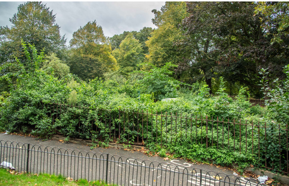
The land behind/above the toilets on Bayswater Road is very overgrown.
