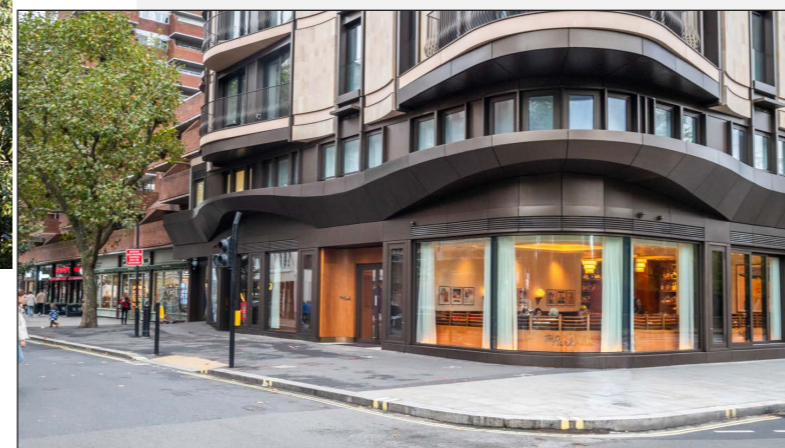
A lamp column at the junction of Queensway with Bayswater Road should be installed by the end of June.
