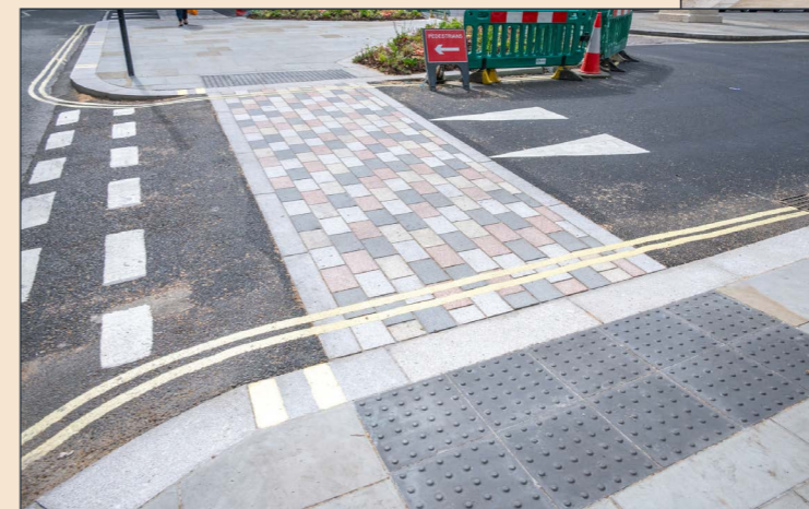
Above and Left - Attractive new stone sets at crossing points, re-aligned kerbs and textured surfaces will deliver safety improvements.
