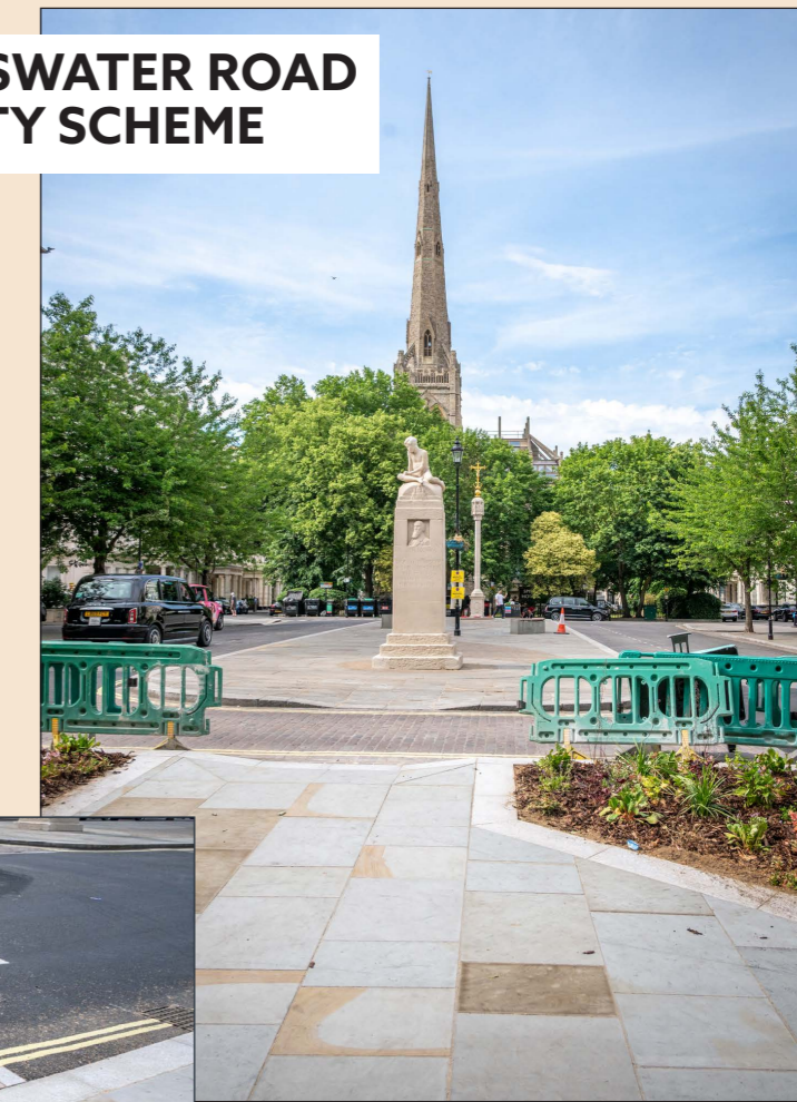
Above and Left - Attractive new stone sets at crossing points, re-aligned kerbs and textured surfaces will deliver safety improvements.
